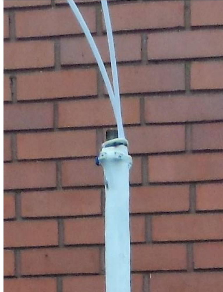
32mm diameter Sock Anchors – tensile capacity 32.7T, shear capacity 21.7T
