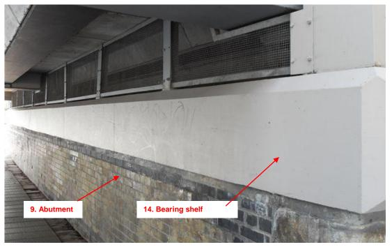
Figure 4: Lea Road Bridge - View showing Abutments and Bearing Plinth/Shelf
