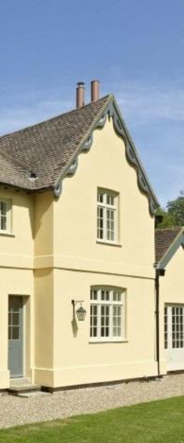
External Wall Insulation
