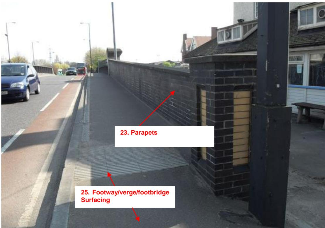
Figure 5: Lea Road Bridge – North East View showing Carriageway, Footway and Parapets
