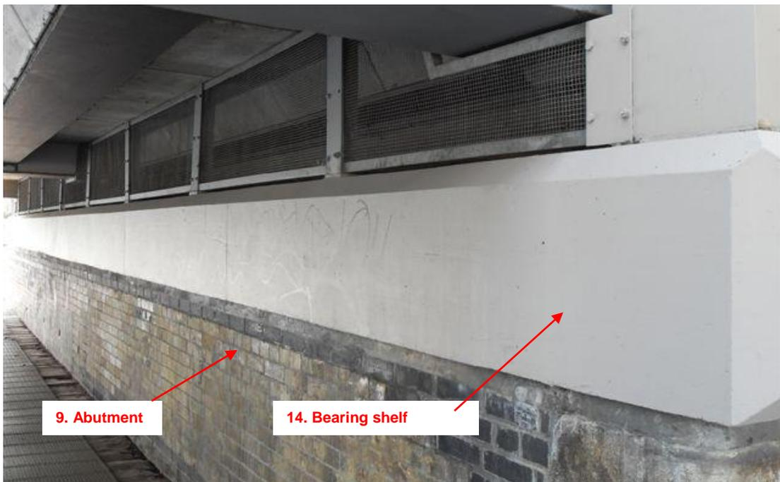
Figure 4: Lea Road Bridge – View showing Abutments and Bearing Plinth/Shelf
