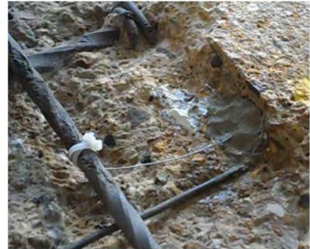
3. Fix anode wire to steel and apply repair mortar
