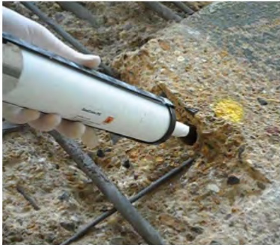
1. Drill a hole and apply PG Mortar
